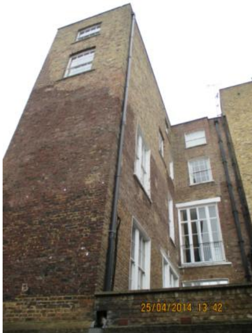
Photograph 3. Rear elevation of 93 Gloucester Place
